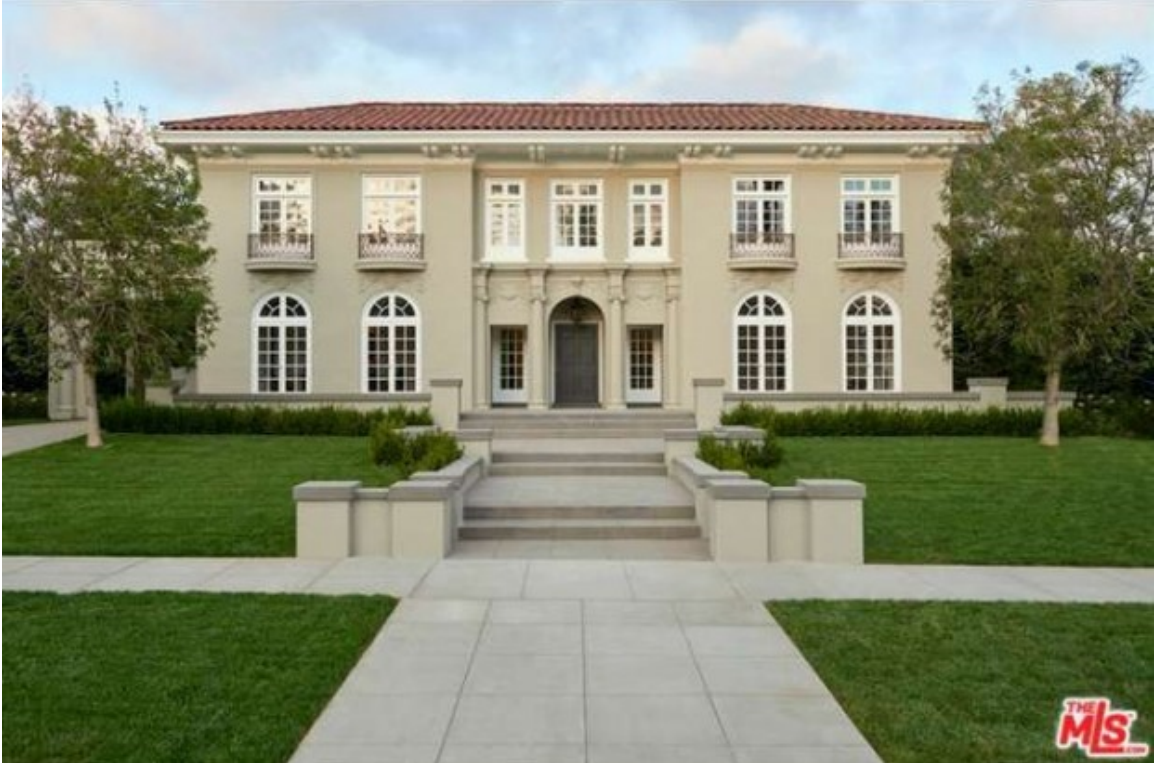
434 South Windsor Boulevard
